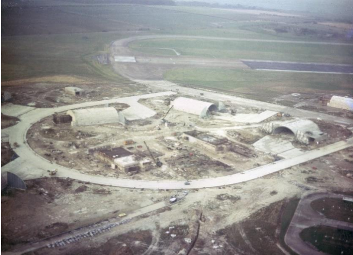
Hardened aircraft shelters under construction at Marham in 1981.
